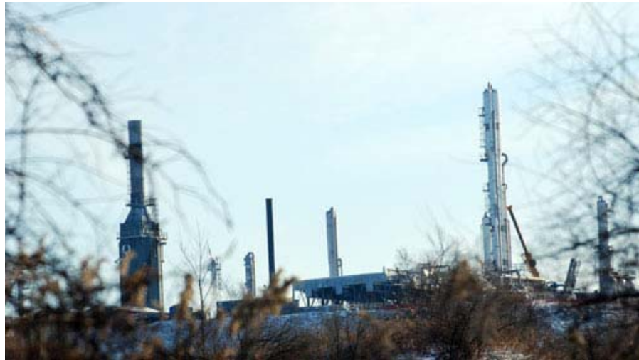
Looking up at the rapidly expanding facility from Rt 519
