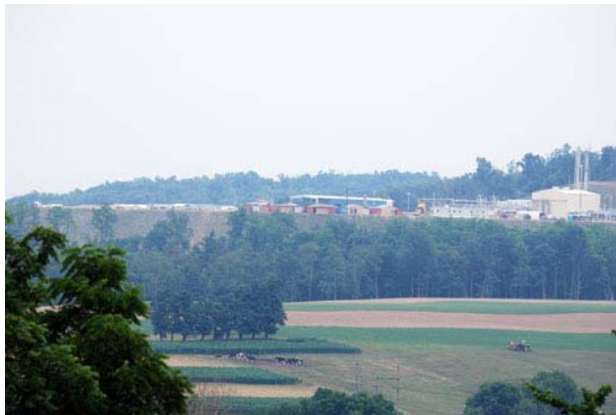
MarkWest's hilltop facility
