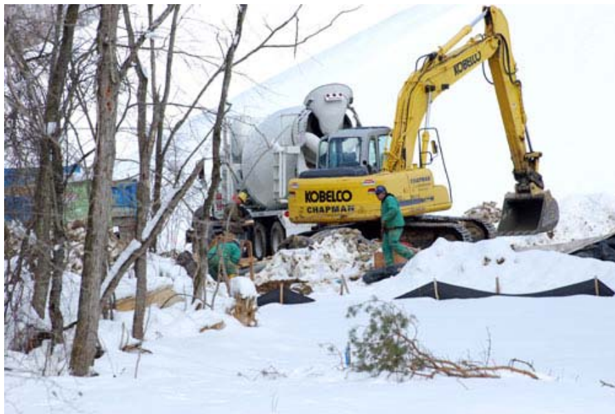
Early 2010 winter construction
