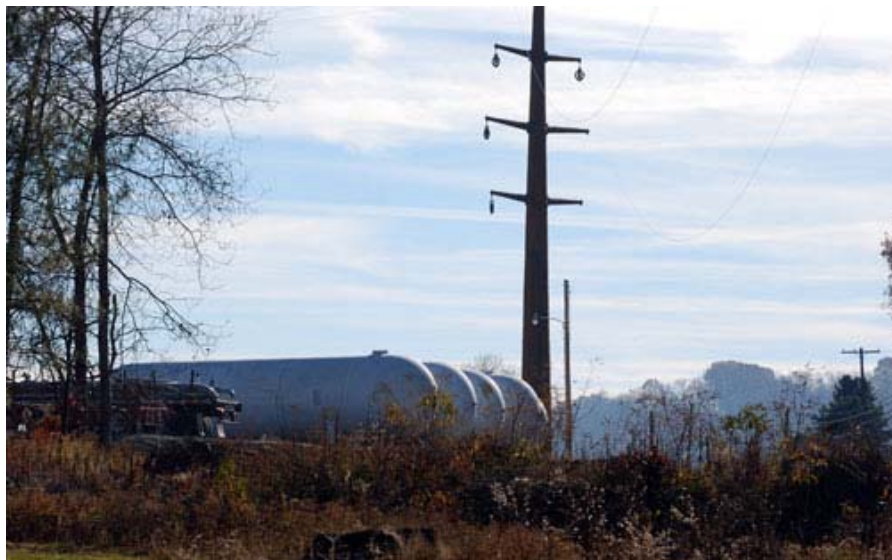
Electric supply towers erected in late-2010 to supply
