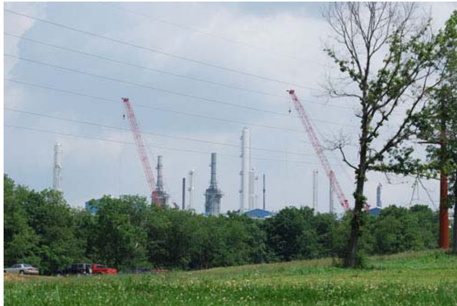
Ongoing construction at the MarkWest plant in July 2011
