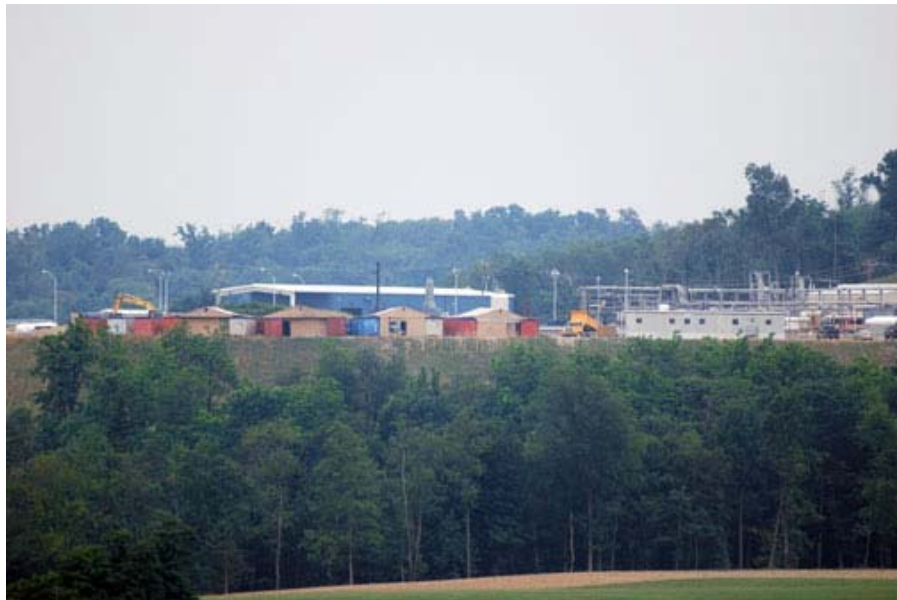
In 2011, MarkWest Liberty plans to expand its cryogenic processing capacity at the Houston plant from 155 MMcf/d to 355 MMcf/d
